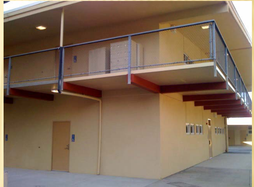
Grossmont High School Building 500 & 700
