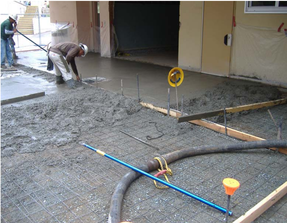
Grossmont High School 800 Bldg - Phase 2B
