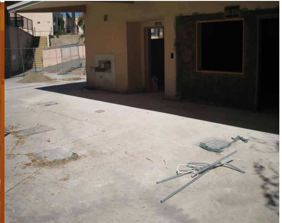
El Cajon Valley High School 500 Bldg - Phase 2B
