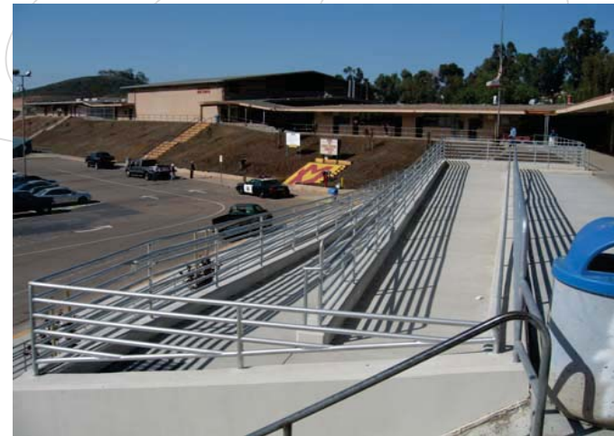
Infrastructure After (Monte Vista High School)
