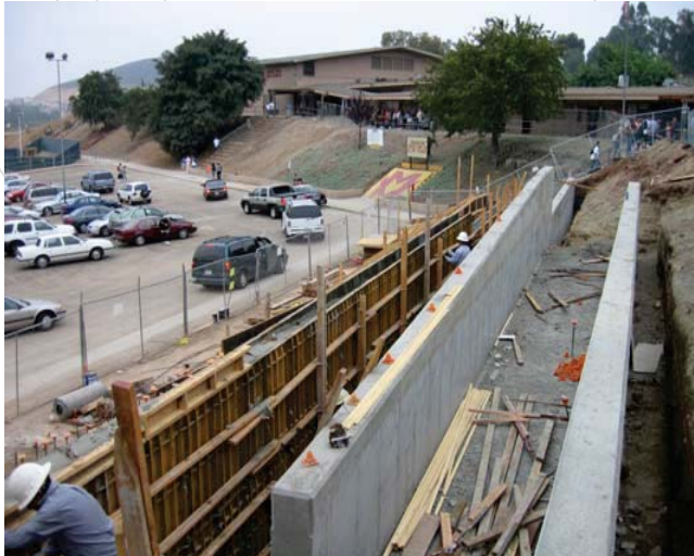
Infrastructure Before (Monte Vista High School)
