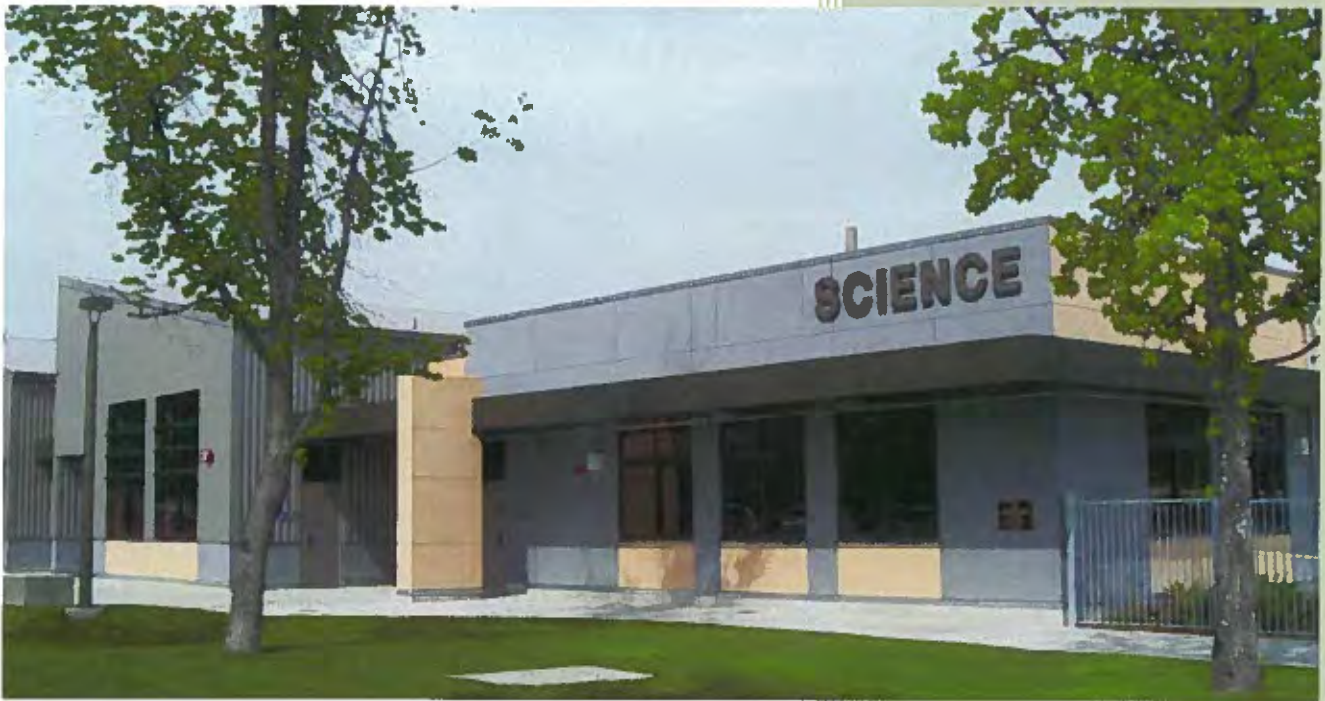
Santana High School – Science Building
