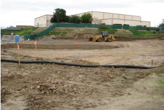
Grossmont High School – Science Building
