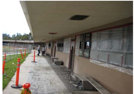
Monte Vista High School – Building 200
