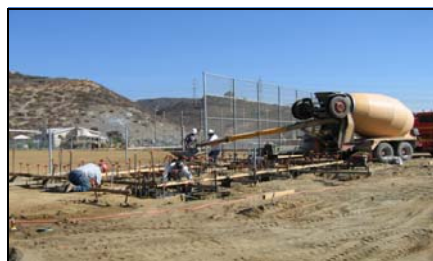
Steele Canyon Concrete Dugout Foundation
