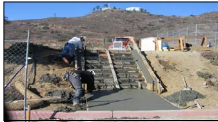
Steele Canyon Steps to Softball/Baseball Field
