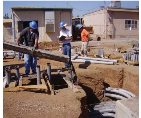
Infrastructure installation at Granite
