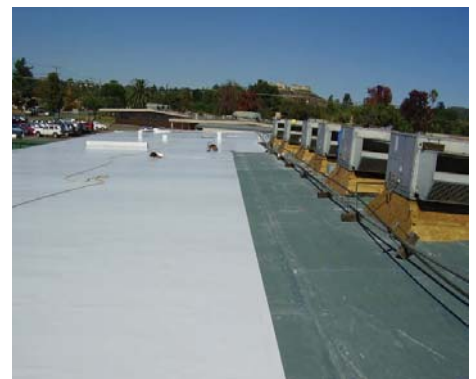
New Roofing Installation
