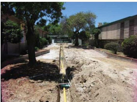
New Waterline Conduit at Helix Charter
