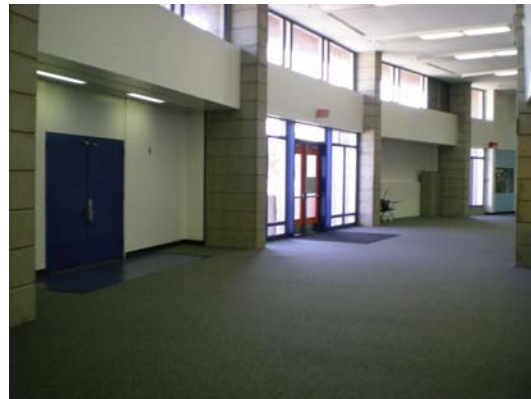
Valhalla High School – Main Bldg 3 rd Floor Main Entrance in front of Administrative Area
