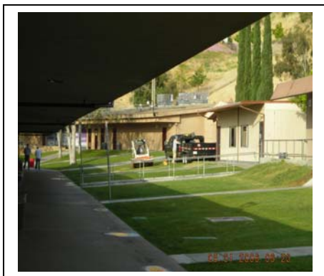
Grading for access path between Buildings 300 and 1200 to begin 5/1/08
