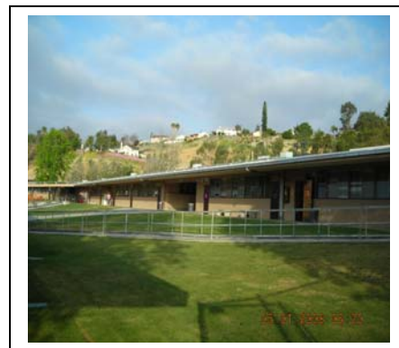
Demo/Abatement at Building 300 to begin 5/7/08
