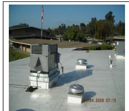
Building 100 Complete Roofing – Pending Walk Pad Installation
