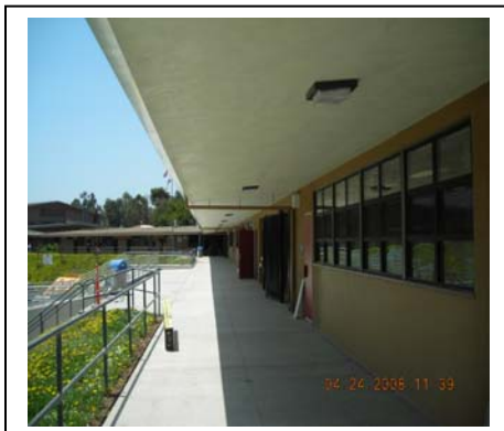
Building 100 Exterior Paint Complete
