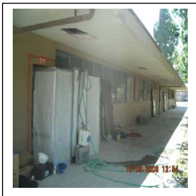
Abatement Ongoing at Building 400
