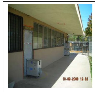
Abatement Ongoing at Building 200
