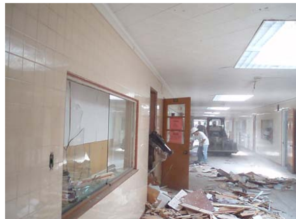
Demo in progress in building 100
