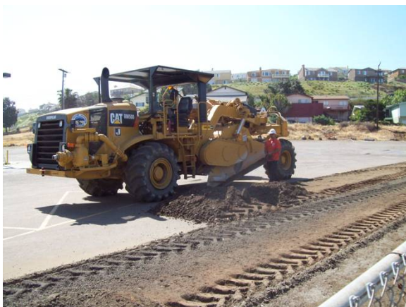
Pulverization in Progress
