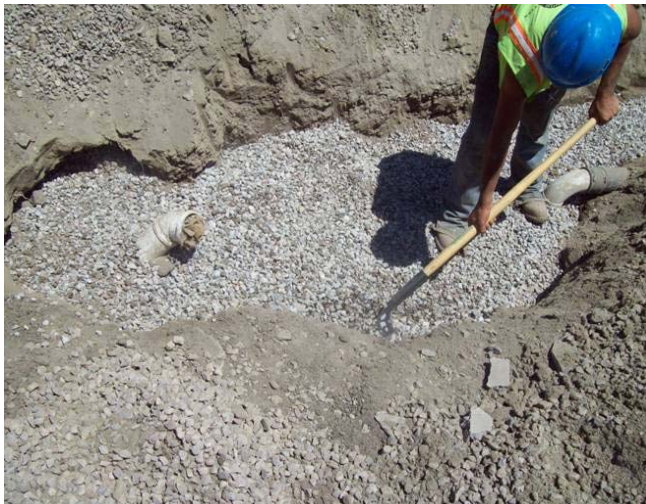
Parking Lot-Storm Drain Installation
