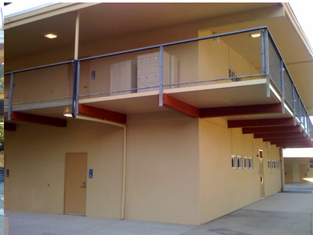
Final Clean and Locker Installation B-700
