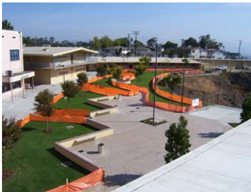
Landscaping complete, remove/replace DG path w/ 'Grasspaver II'
