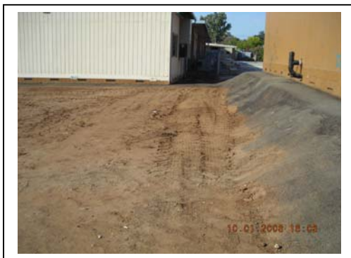
Grading of dirt lot which was occupied by former live on.
