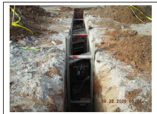
Shoring for fire water trench.
