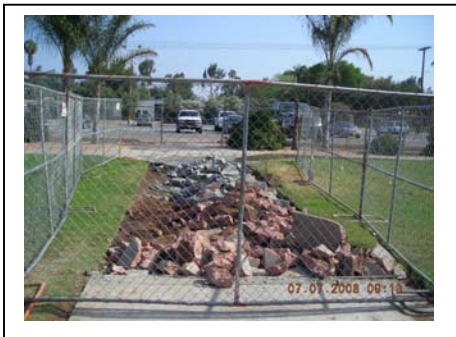
Concrete demo north of gym.
