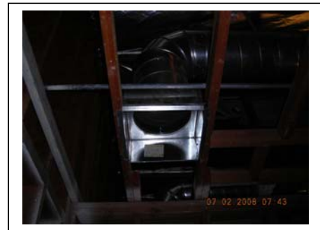
Exhaust fan installation at 120 RR.
