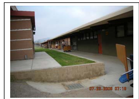
Moving out of 800 Building.
