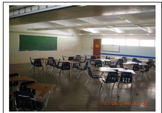
Before Interior Classroom at Building 1000
