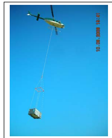
Flying in HVAC Units for Building 800
